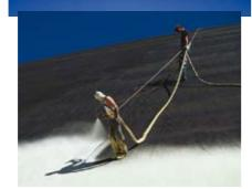
With volume solids of 64% Hardtop Flexi is more friendly to the environment with low VOC emissions. That makes it popular with applicators too. Plus, it can be applied up to 150µm DFT in a single coat bringing benefits for yard and owner – fewer coats are needed, reducing downtime and application time.
