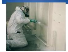
Fast drying is a primary benefit with Hardtop Flexi, particularly when time is short and costs of downtime are high. Surface dry in just 90 minutes at 23°C and in only 3 hours at 10°C means project progress can be maintained with minimum delay combining with the benefits of fewer coats to maximise efficiency.
